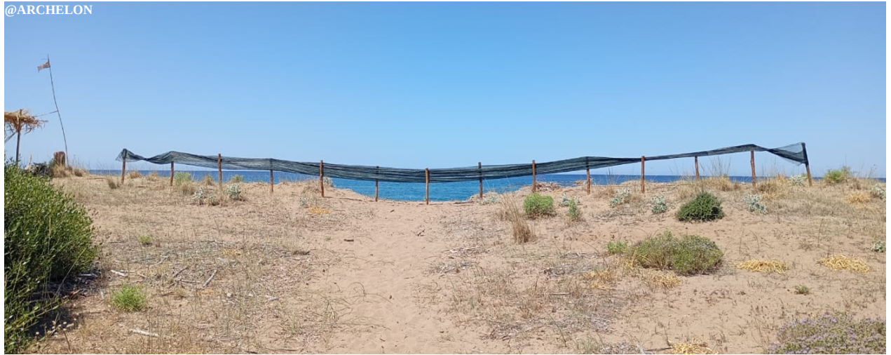
Fig. 3b | Temporary fencing installed as part of a pilot dune restoration action between Agiannakis and Elaia, June–July 2026.
