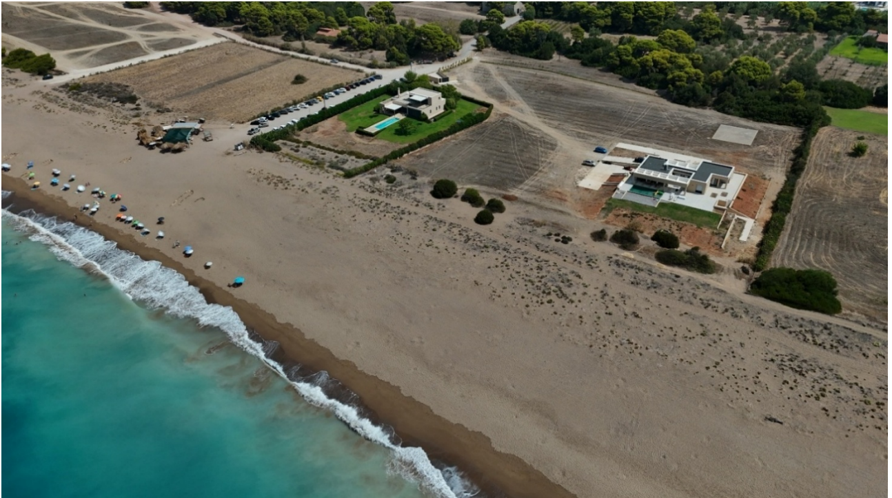
Photo 5a: Agiannakis, 22 August 2025 – The construction of these villas was approved without the impact on the sand dune habitat to be assessed.
