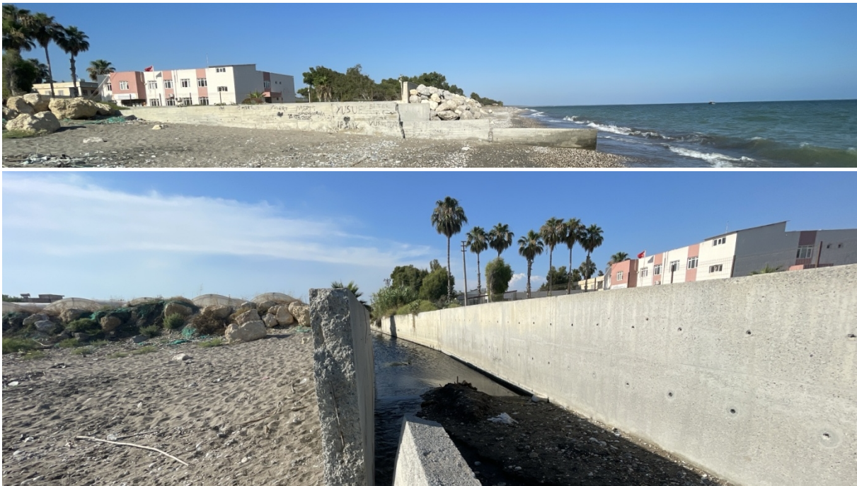
Figure 14 The concrete canal next to the school and the barriers protecting the school from waves.
