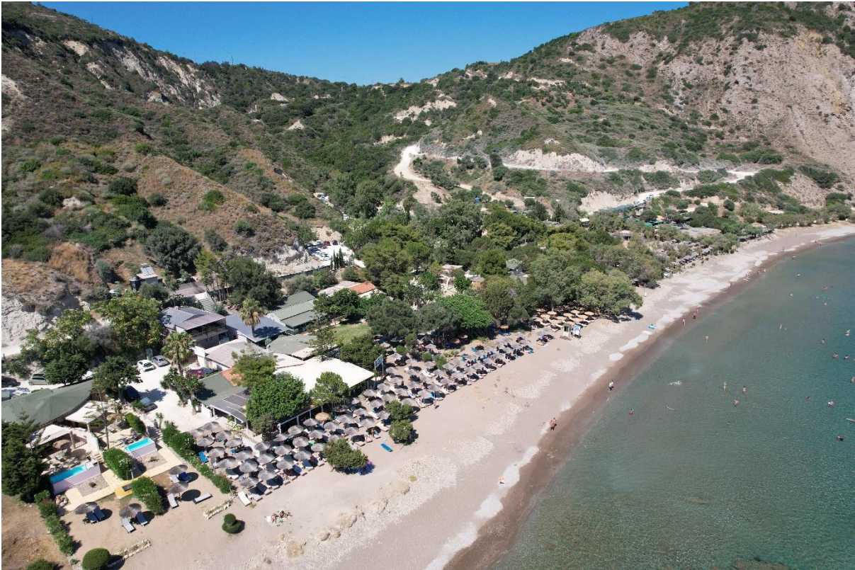
Fig. 3 | Dafni, 30 June 2025: Natural sand dune system destroyed. The situation remains unchanged. All the buildings seen in this figure are illegal.
