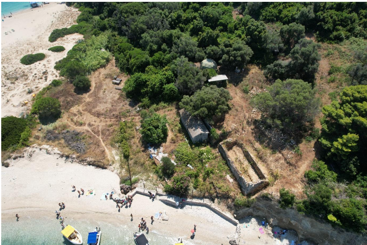
Fig. 10 | Marathonisi construction area. The construction area in Marathonisi island seems unchanged since the temporary stop work order was issued in 2025.
