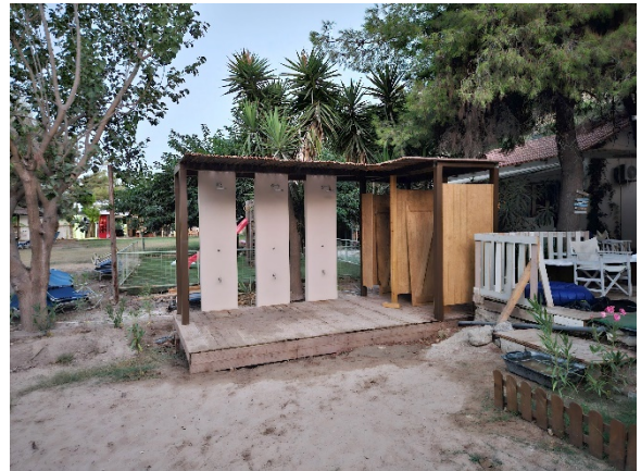
Photo 4d: Newly built shower facility (Daphni, August 2025)
