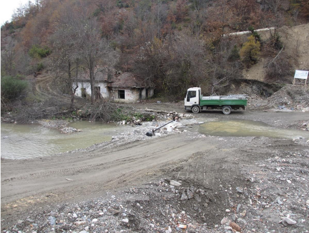
Picture 1. LPHPP construction on Tresonecka River
