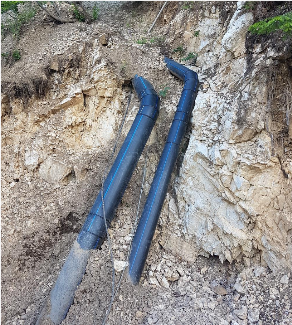
Picture 4. LPHPP construction on Kakaacka River
