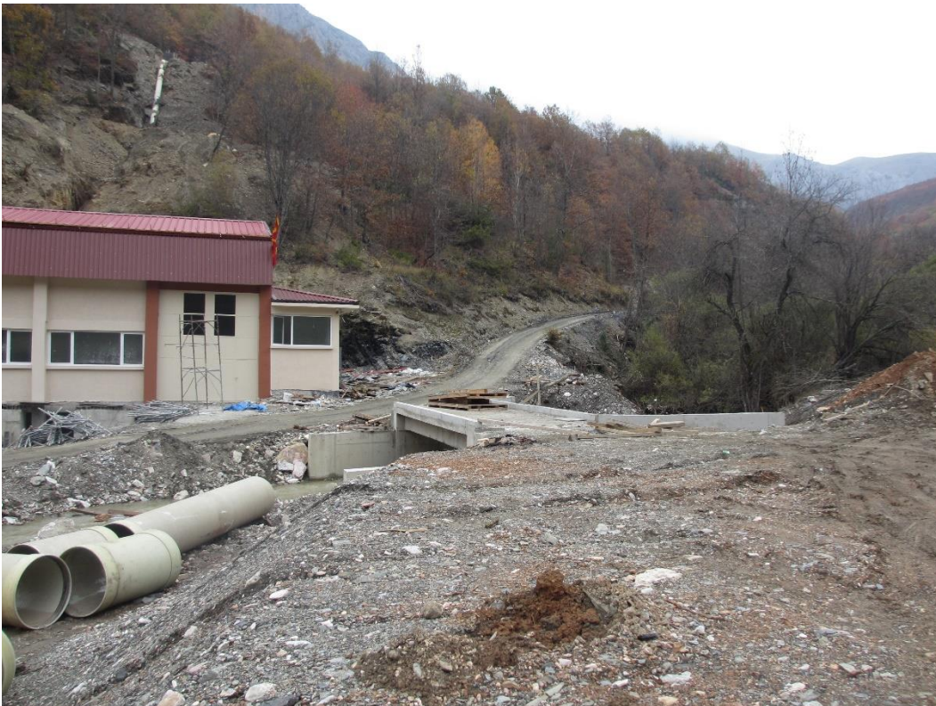
Picture 2. LPHPP construction on Tresonecka River
