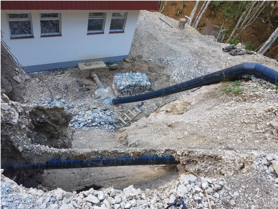
Picture 3. LPHPP construction on Kakaacka River
