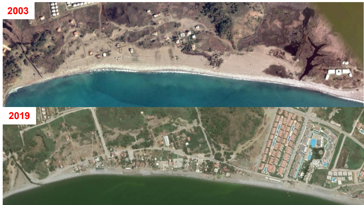
Fig. 2. Fethiye SPA. Çalış Section B. Google Earth 2003 – 2019 satellite imagery comparison shows the continual coastal build-up, planting of sandy area and occupation of nesting beach, in conflict with Recommendations. Note that the sandy area (nesting zone) has been occupied and, in most parts, only the pebbly zone near the waterline is development-free.
