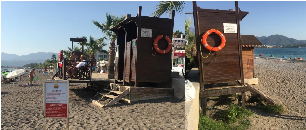
Fig. 12-13. Fethiye SPA. Çalış. Section A. Showers cabins remain on the beach and water leaks directly onto the nesting zone. Note vegetation growth due to water runoff (right).
