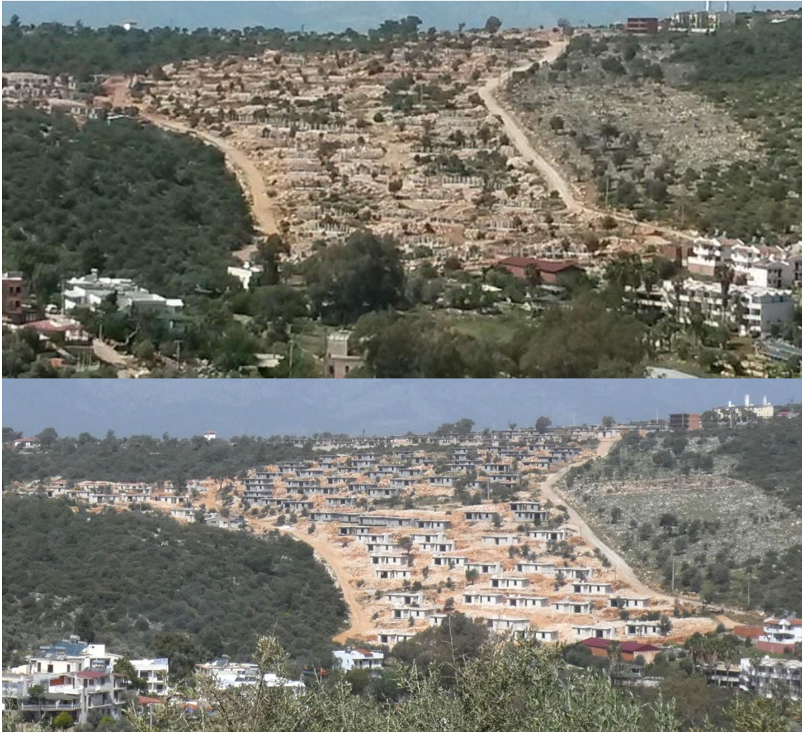
Fig. 28-29. Patara SPA. 3 rd Degree Archaeological Site. Top: June 2016. Bottom: April 2018. Construction work continues for approx. 310 buildings in different stages of construction.
