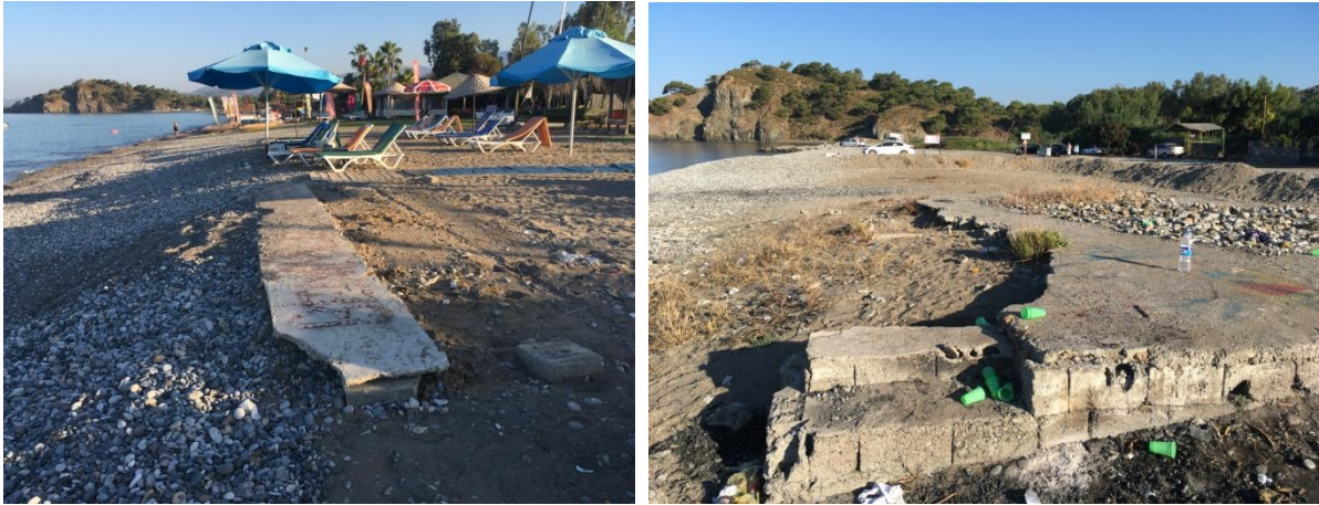
Fig. 3-4. Fethiye SPA. Çalış Section B. Concrete platforms on nesting beach (left: new in front of Spor Café; right: existing abandoned cement platform).
