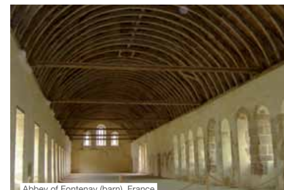
Abbey of Fontenay (barn), France
