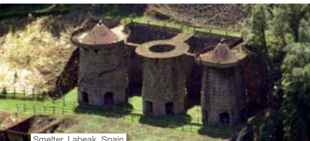
Smelter, Labeak, Spain
