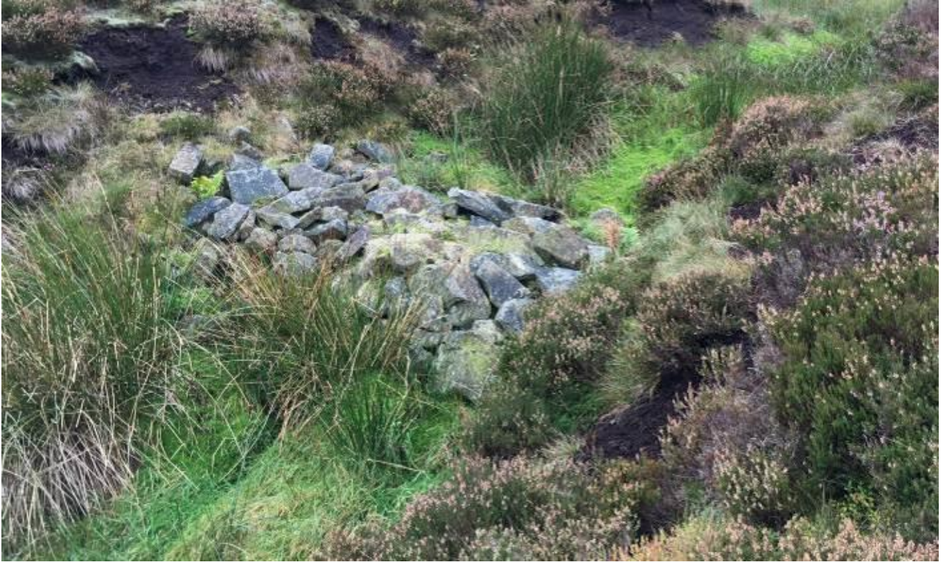
A stone dam in process of coverage by grass (Photo: Anna Badcock PDNPA)
