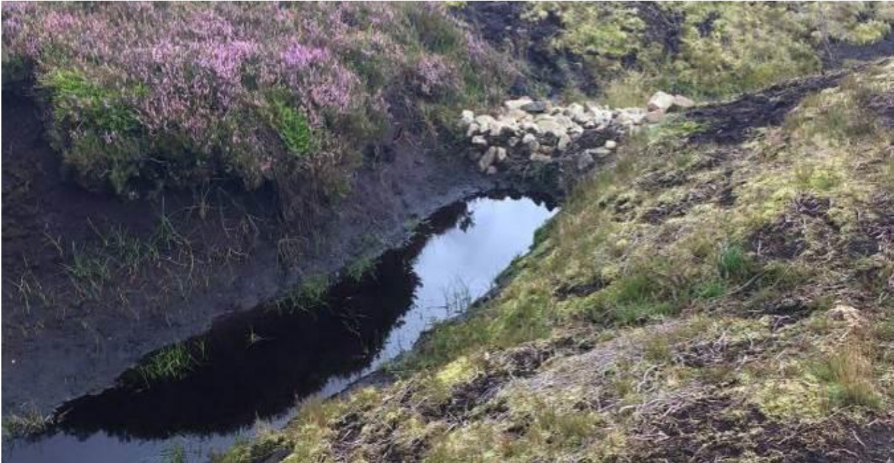
A stone dike against the erosion of blanket bogs (Photo: Anna Badcock PDNPA)
