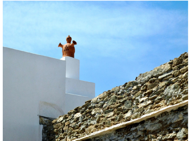
Top part of the clay chimney in use on Sifnos island © European Route of Ceramics
