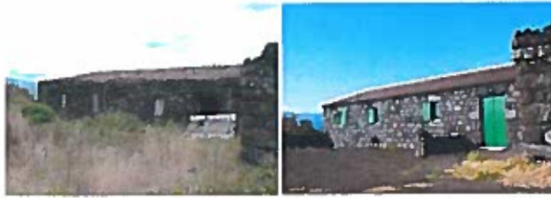
Reconstruction of dilapidated building (still)
