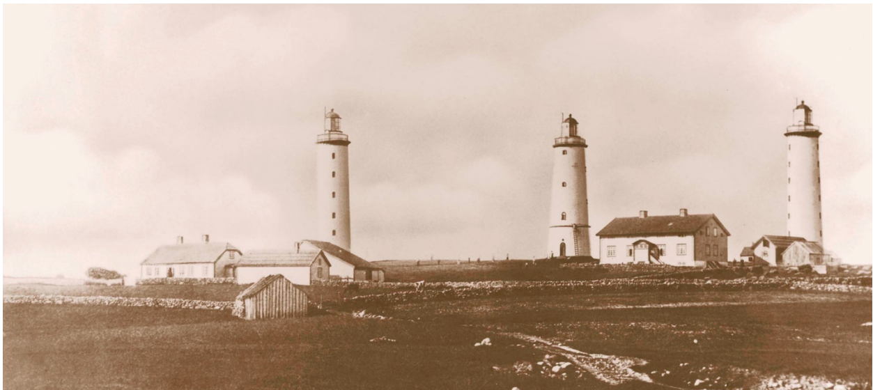
The Lista Lighthouse Station had three towers in the period from 1853 to 1873. Photo: Listafyr.no
