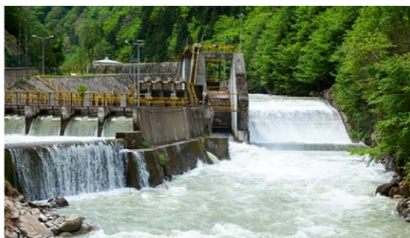
Small hydropower plant
