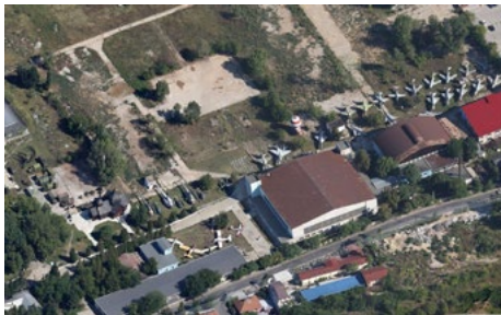
Urban renewal is the rebirth of the extinct art of creating and re-creating places or essentially, the reorganization of built
