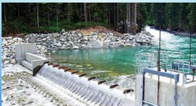
Photo 6. Small HydroPower Plant in Republika Srpska, Bosnia and Herzegovina Source: https://infobosnia.com/central/central-presudom-slobodan-razvoju-energije-grebene-iz-izvora-hidroelektrany/24226
