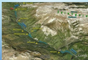
Image 2. Map of the small HydroPower Plants on the River Neretva, Bosnia and Herzegovina Source: https://www.aj.gov.ba/central/central-za-ocuvanje-narodno-parkova-i-narodno-parkova
