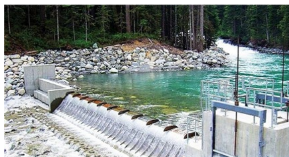
Small hydropower plant in Republika Srpska, Bosnia and Herzegovina
