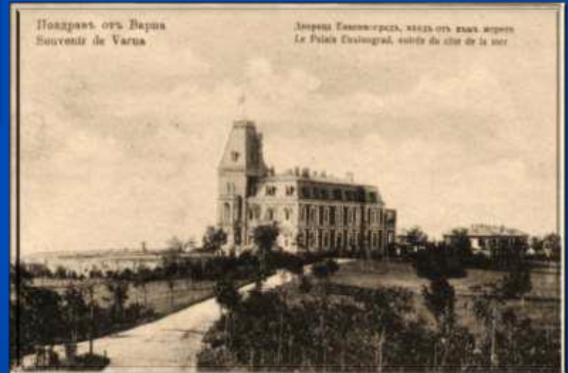
□ View of the palace and garden
