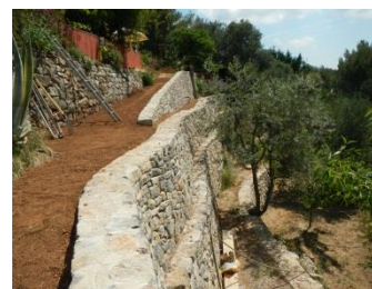
Fig. 59. Toulon (Var), France. Retaining wall built by Albert Porri, waller.
