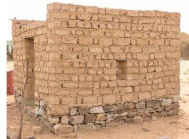
Fig. 68. Foundations and base of a new mud-brick house, Chinguetti, Mauritania.
