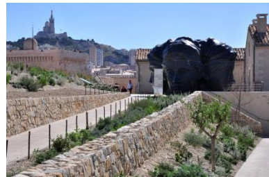
Fig. 47. First prize in the 2014 Victoires du Paysage landscape competition in the “Urban Garden” category: Jardin des Migrations, Fort Saint-Jean, Marseille, France. Design: APS, Valence. Construction: Les Murailleurs de Provence, trainers for the Acta Vista work experience scheme.
