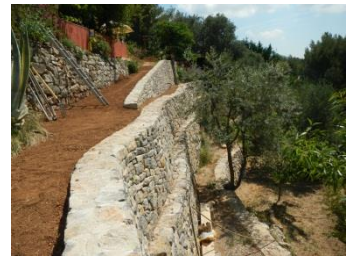
Fig. 59. Toulon (Var), France. Retaining wall built by Albert Porri, waller.
