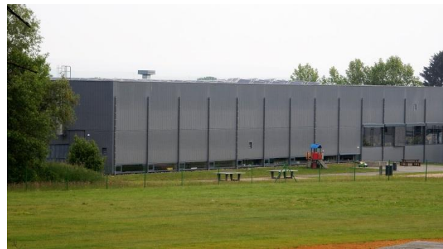
Joint-owned solar panels installed discreetly on a sports hall in Beckerich (L)
