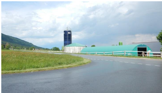
Biomethanisation plant in the foothills of the Jura (CH)
