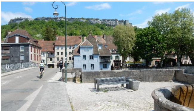
The bridge over the River Loue, Ornans (F)
