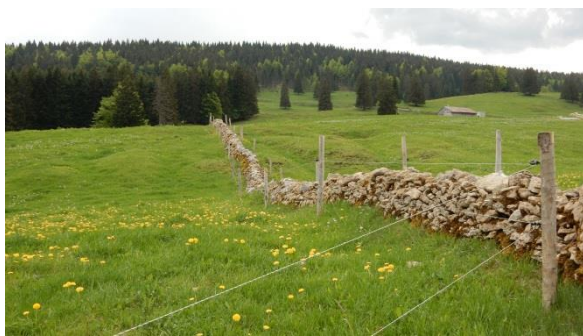
Recently restored stone walls (F)
