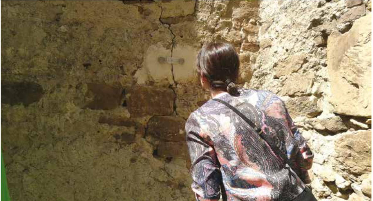
A marker for recording evolution of structural cracks on the walls of the fortified church of Alma Vii. While restoration works are, for now, exceeding the capacity of the community to undergo, the condition of the fortified church is strictly monitored and maintained.
