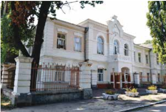
The Mihai Eminescu High School Soroca, Republic of Moldova, currently abandoned, was evaluated for rehabilitation and reconversion to new educational uses
