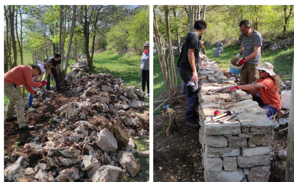
Traditional drywall construction techniques, Livno 2024 ©Zvonimir Malbaša; 4 GRADA DRAGODID
