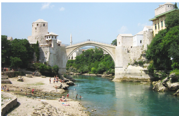
Mostar Bridge, ©Wikipedia
