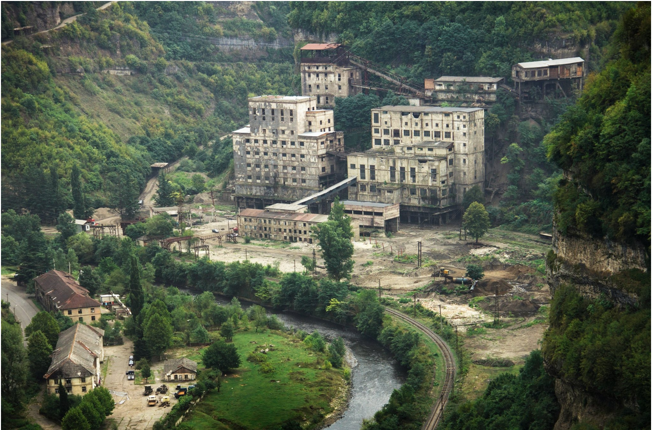
Caption 3: Central enrichment plant, 2016
