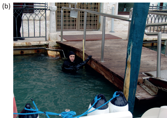
1.- The sea level has reached and submerged the doorstep. (a) A view during maintenance works. The floor has been raised 1 m and the lower part of the door has been bricked up and used to host sewage drainage pipes (photo D. Resini, courtesy INSULA, Venice). (b) The Frogman of the State Police is taking measurements standing on the bottom step of the sea stair, that now is fully submerged; a wooden walk-way was built to reach the door.
