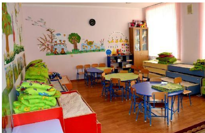
Kindergarten renovation in Molovata, Dubasari
