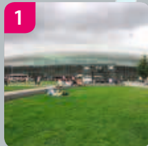
1 Rail station Place de la Gare
