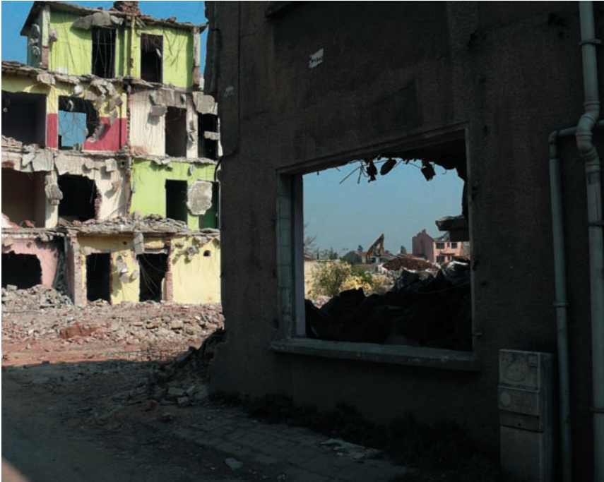
Demolition of Sulukule – Turkey.
