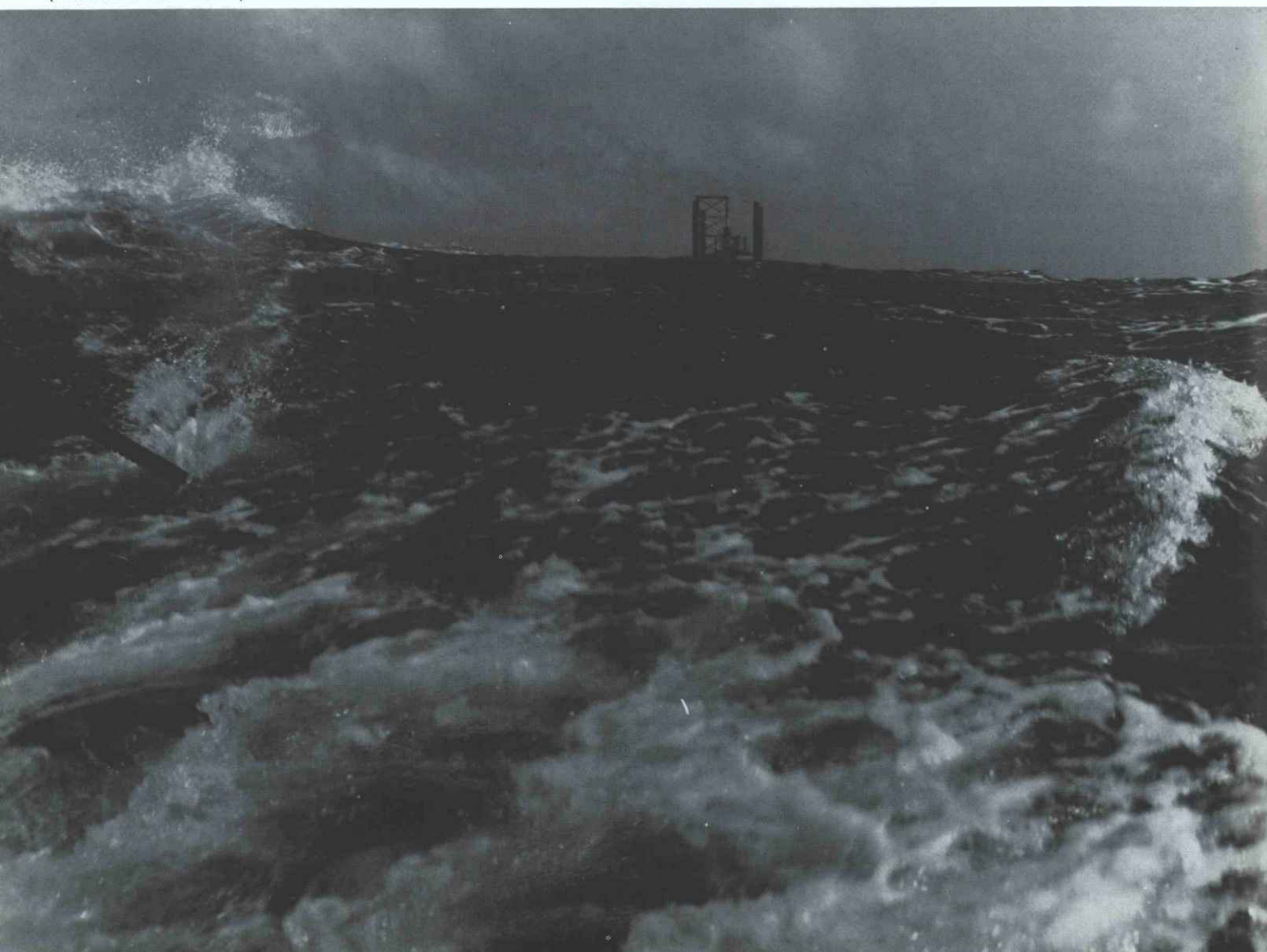
A drilling platform arrives over the horizon - who rules the ocean floor and its resources? (Photo C. van der Meulen)
