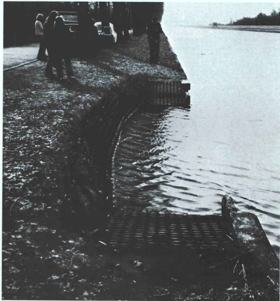
It is often possible to avoid accidents like drowning — construction on canal banks in The Netherlands permitting game to mount the steep inclines
