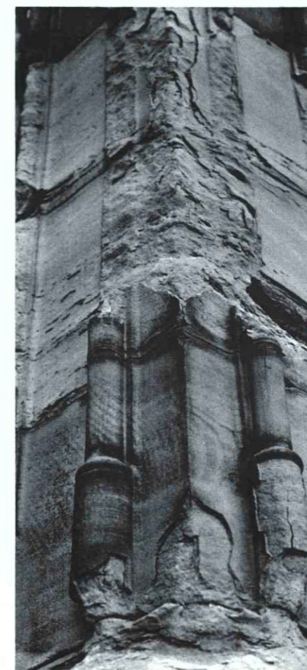
Pollution has also aggravated the natural decay of many irreplaceable monuments, such as the Strasbourg Cathedral.
