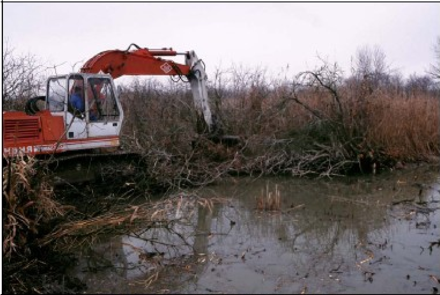
Picture 9: Process of cleaning of former bricklayers' holes of Teglaz
