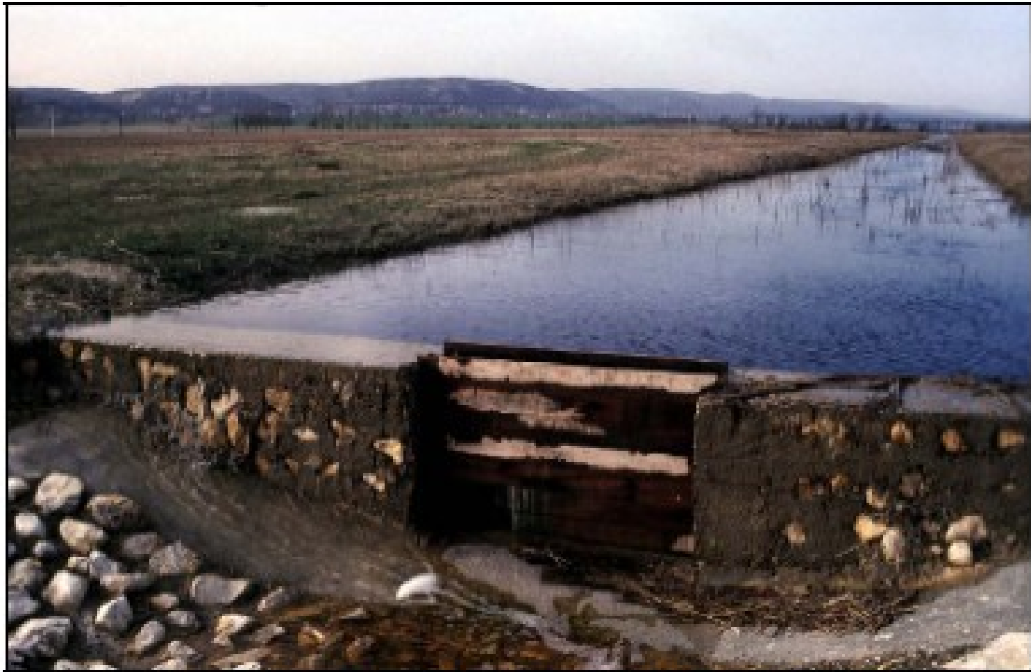
Picture 7: Inhibiting facility (sluice) for preservation of the available water
