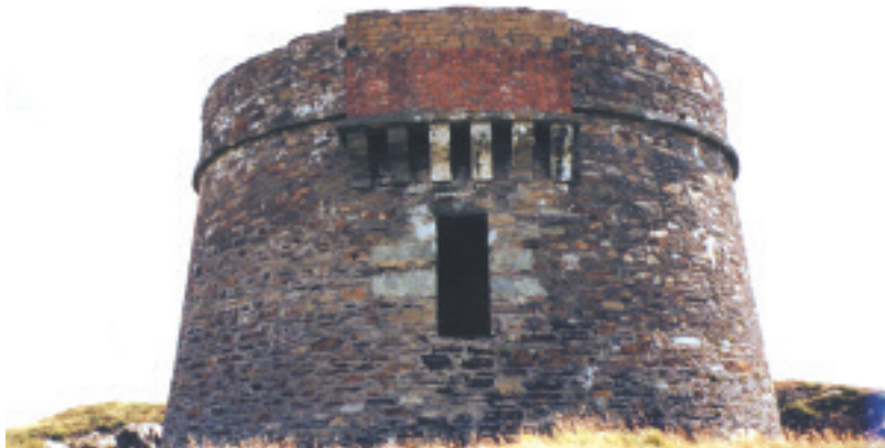
Plate 2: View of Martello Tower on Clochann Hill
