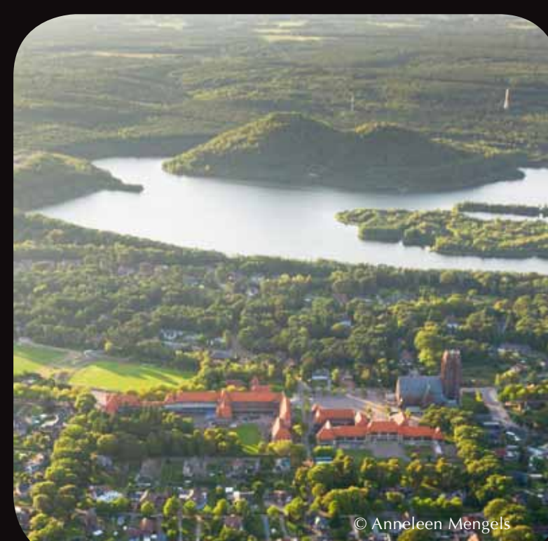
Aerial view of one of the garden cities with typical street pattern and tree plantation prescriptions, and coal tips of belonging mining site in background.
