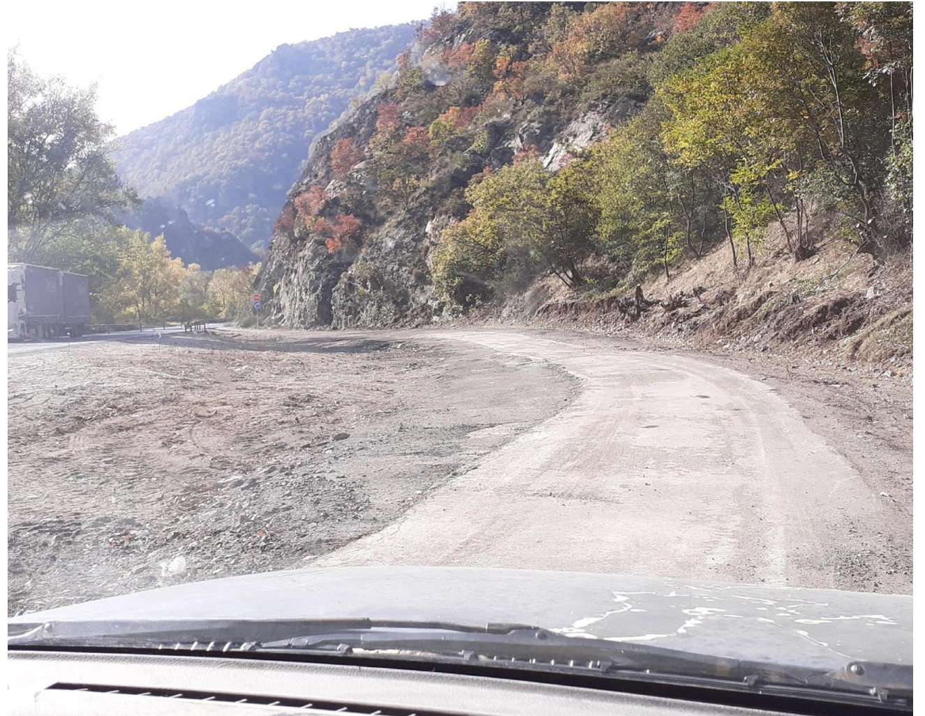
Clearance of vegetation in preparation for asphalt coverage, October 2022
