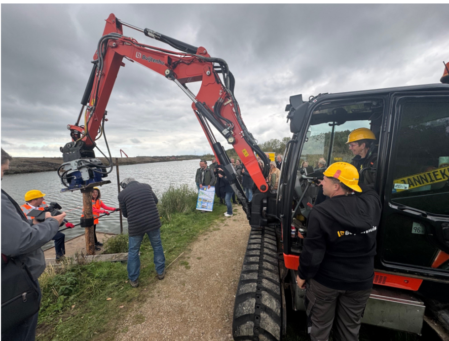
Figure 2. Start of work in the Oostvaardersplassen Almere gate area
