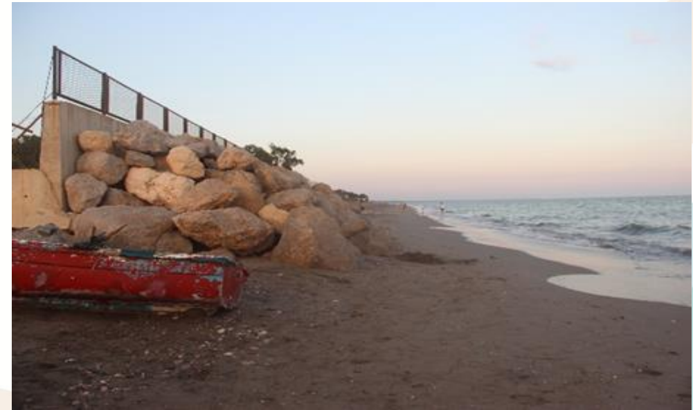
Arbitrary use of boulders and concrete/cement Structures.
