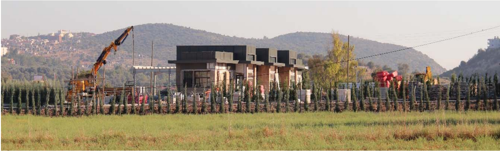
Construction of “welcome centre” in the archaeological site behind the beach
