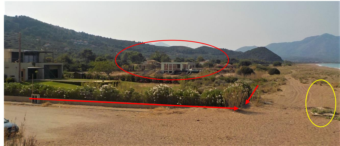
In Agiannakis a new villa (red circle) and a shower (yellow circle) construction on the beach, and further planting and maintain of introduced alien plant species
