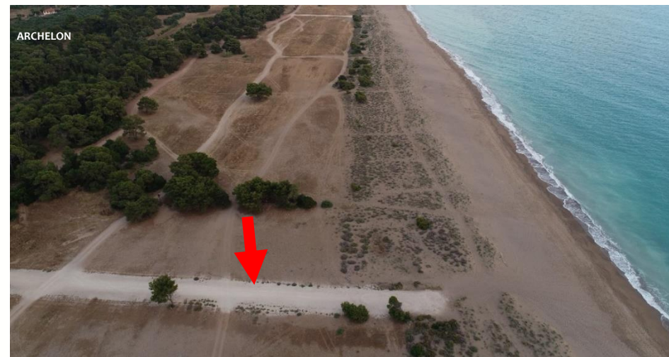
One of five illegal roads constructed in 2012, has not been restored to date
