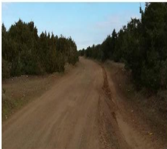
Current natural dirt road
