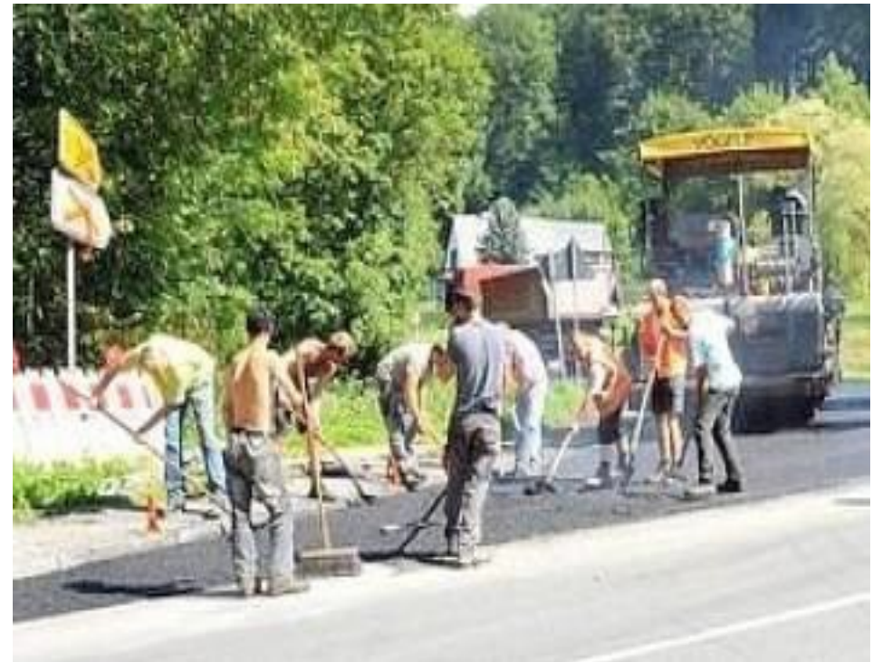
Germany: Rural road construction: 'typical' male work.
