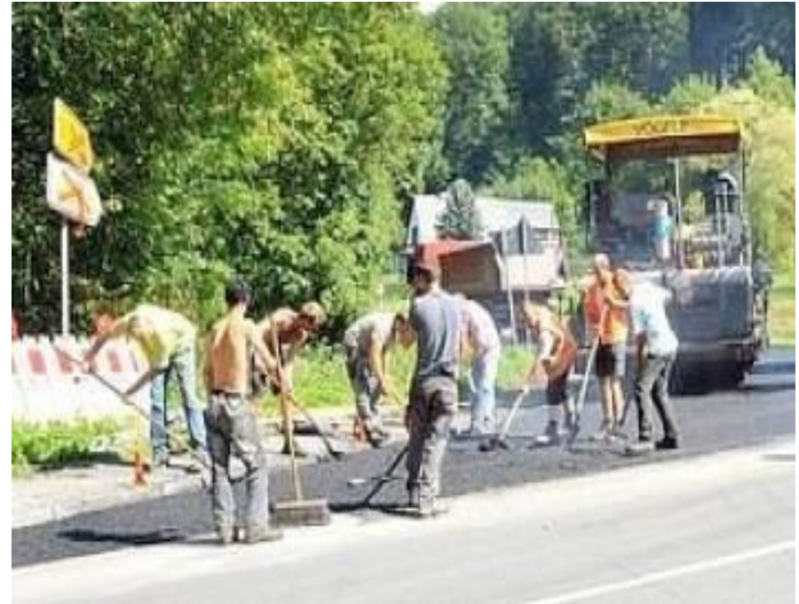
Germany: Rural road construction: 'typical' male work.
