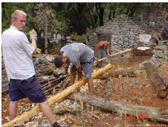
Scandinavian students preparing timber for reconstruction of a roof in Dragodid hamlet in 2002 © 4 Grada Dragodid
