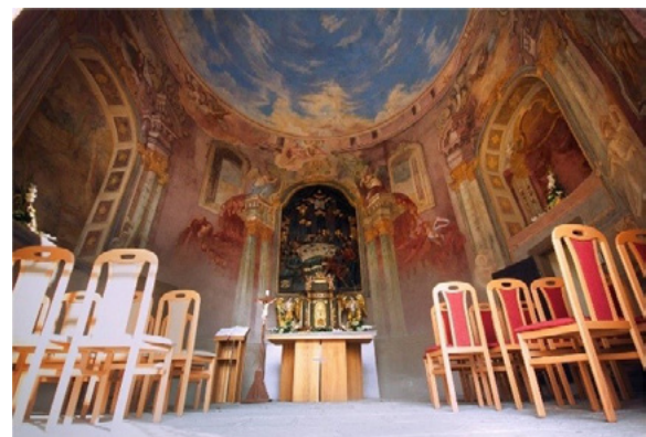
Lower Church – state of the interior after restoration works. © The Calvary Fund archives
