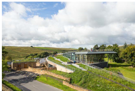
View of The Sill: National Landscape Discovery Centre on Hadrian's Wall. © Northumberland National Park Authority
