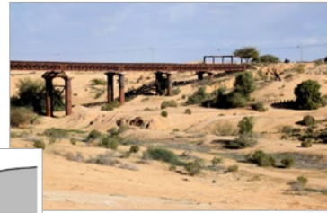
Remains of an old British railway bridge over Ofakim stream
