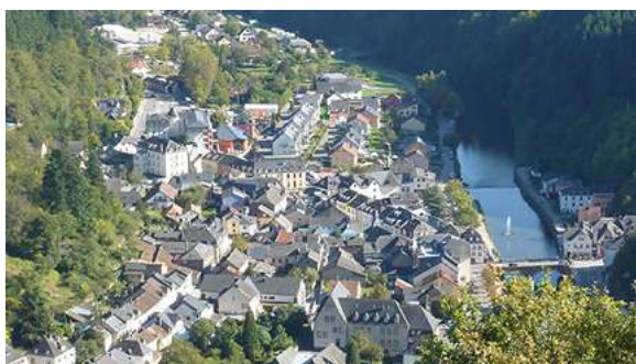
Figure 27. Integration of new buildings in Vianden, Luxembourg
