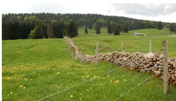
Figure 26. Recently restored stone walls, France
