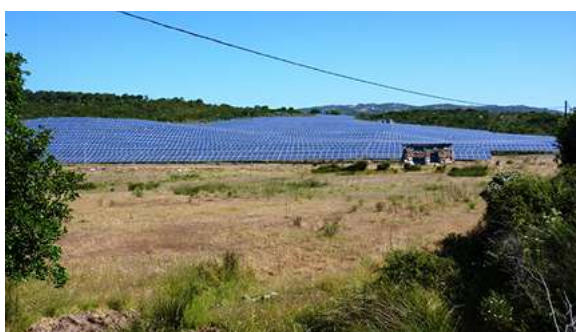
Figure 17. Photovoltaic field beside a motorway, Portugal
