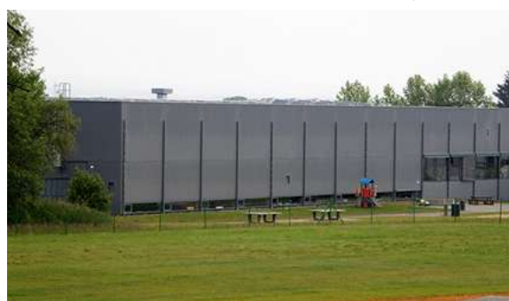
Figure 16. Jointly owned solar panels installed discreetly on a sports hall in Beckerich, Luxembourg
