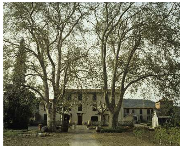
Figure 83. Plane trees framing a traditional farm building transformed into a house (Photo: R. Ambroise)
