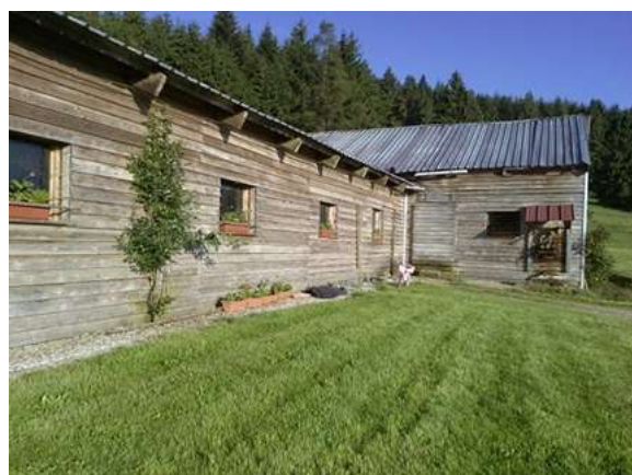
Figure 91. Weatherboarding and climbing plants on a building in France (Photo: R. Ambroise)
