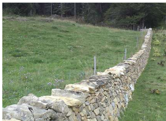
Figure 22. Stone boundary wall (Photo: R. Ambroise)
