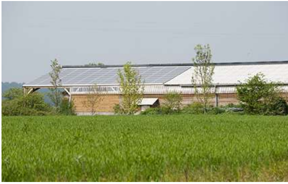
Figure 53. Solar panels on shed roof (Photo: P. Xicluna / Ministry of Agriculture, France)
