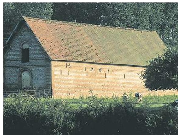
Figure 14. Stone and brick barn in Normandy, France (Photo: R. Sauvaire)
