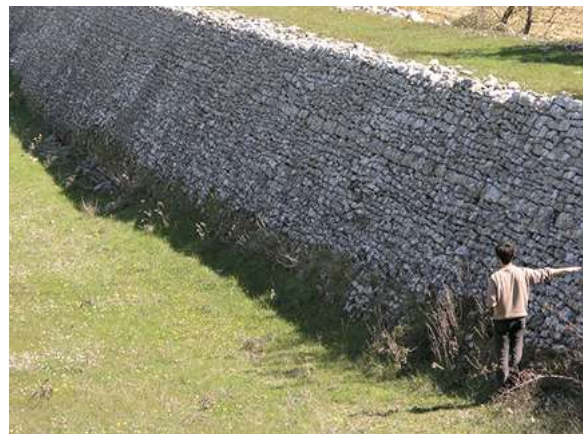
Figure 100. Double-skinned dam (restanque) barring a valley, Switzerland (The waller is pointing to his work)
