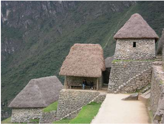
Figure 2. Building with available materials: stone, wood, thatch. Reconstruction at Machu Picchu, Peru (2007)
