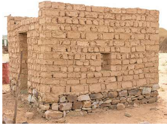
Figure 69. Foundations and base of a new mud-brick house, Chinguetti, Mauritania
