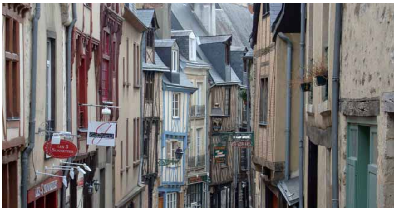
Le Mans, France: a patiently constructed mediaeval framework
