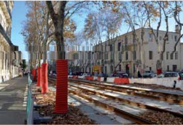
Track extension work, line 3, Montpellier, France
