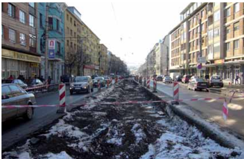
Track modernisation work, line 101, Cluj-Napoca, Romania
