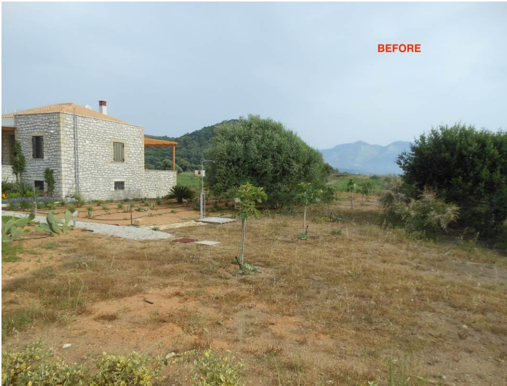
Picture 2. A new fencing construction around the summer house in Vounaki area.
