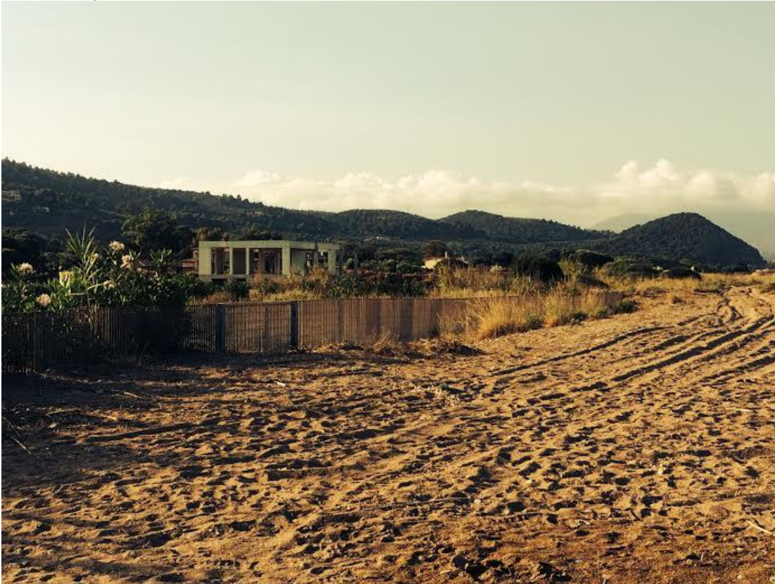
Picture 3. Vehicle tracks are a daily occurrence. No building demolition protocols have been executed in the area yet.
