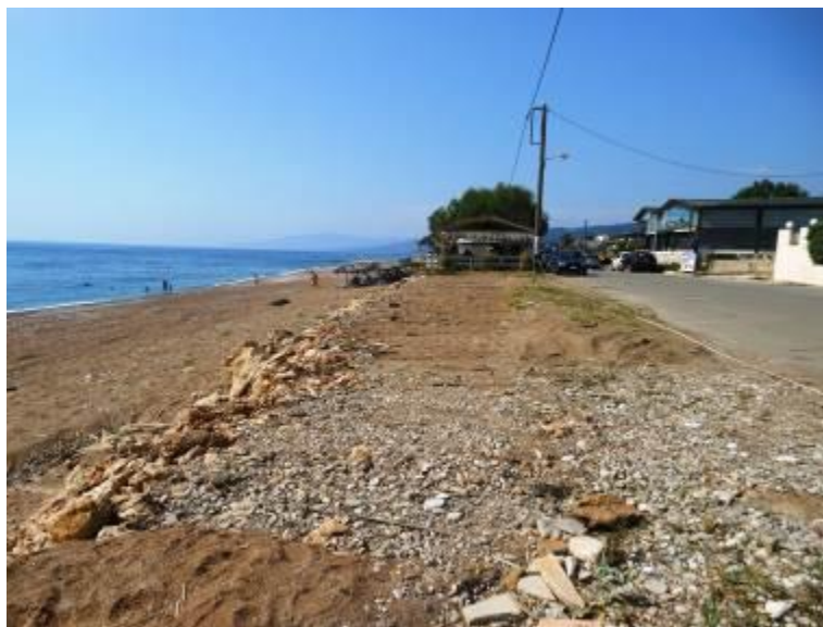
Photo 8: The part of the beach after the demolition of the illegal platform of Messina Mare hotel.
