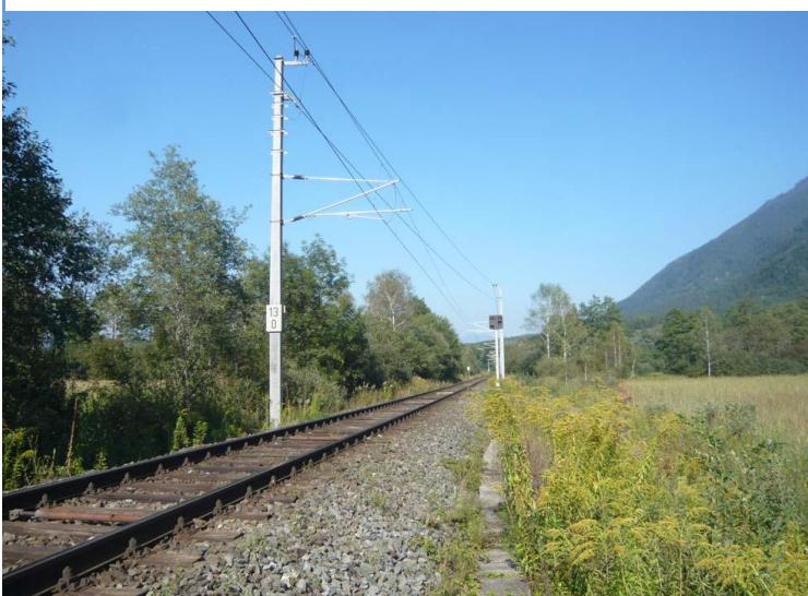
*Picture 4:* Railway power line run by the Austrian national railway company.
