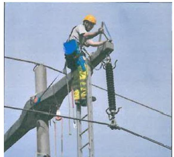
*Picture 3:* 110 kV power line from Schaan to Eschen. "Metallic triangles" were installed in 2013 to hinder birds from landing.
