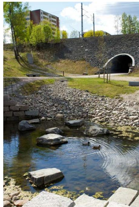
The actual underpass is a 40 metres long steel pipe (culvert) dug down beneath the railway tracks. The underpass was named the Haugen Gate after a naming contest.
